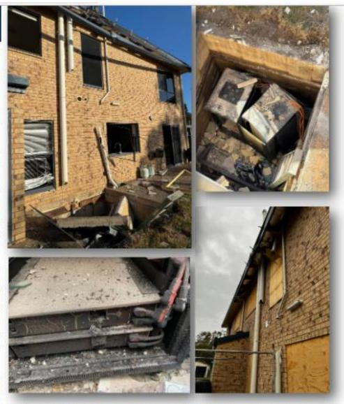
Damage from the lithium battery explosion at my Aunt and Uncle's house. They moved their bedroom to the other end of the house, as it was right above the explosion and sustained significant damage.
